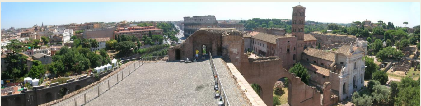
An example of accelerometer monitoring on Rome Monuments
