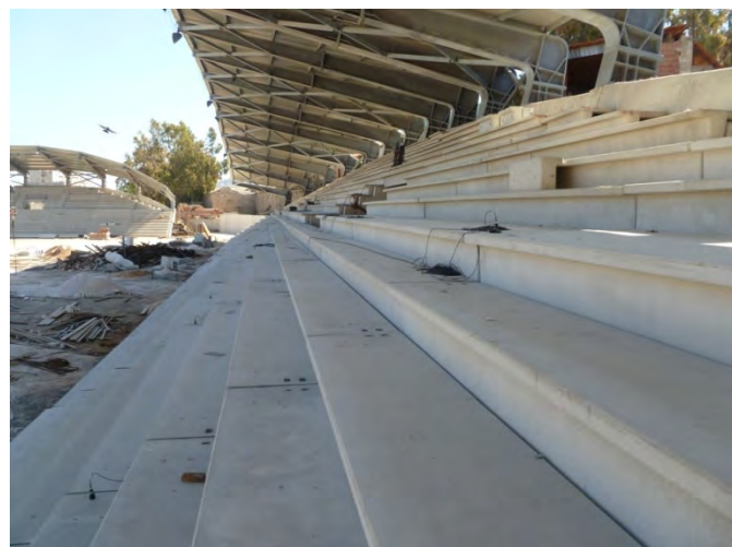
An example of accelerometer monitoring on a football stadium
